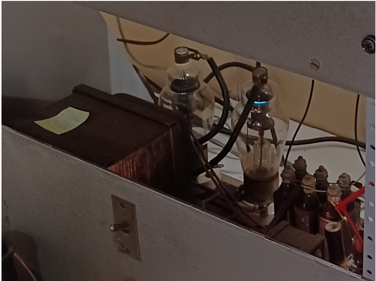
Closeup of the two 866's in the Power Supply (rack bottom deck)
